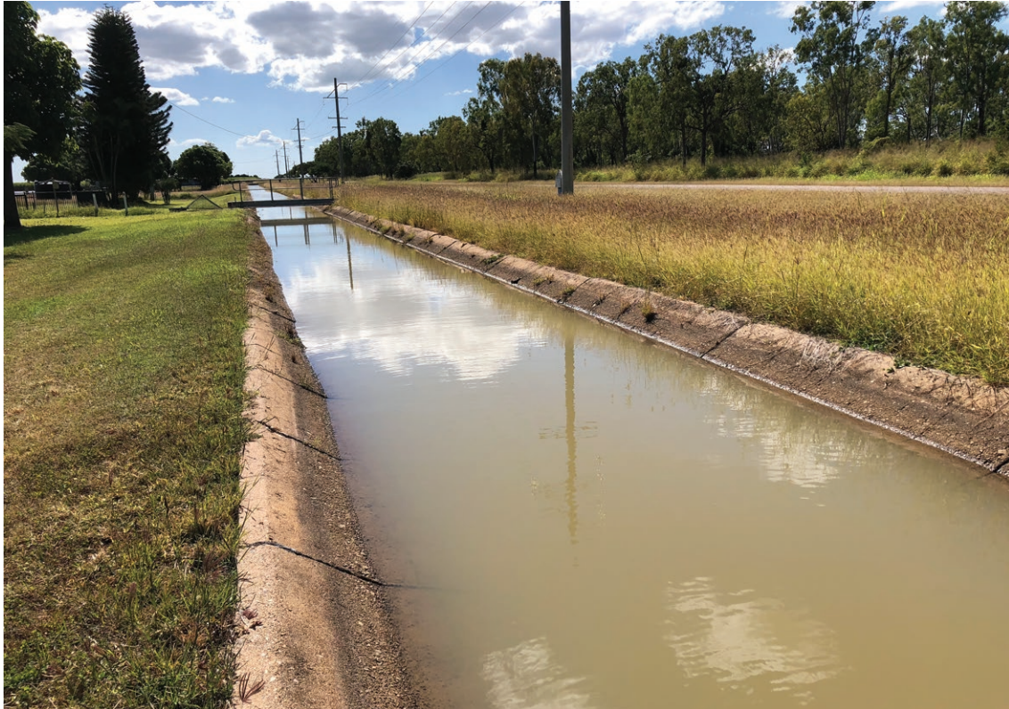
Figure 5. A concrete-lined agricultural water channel.
